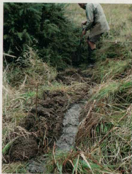
The trench above the headcut.
