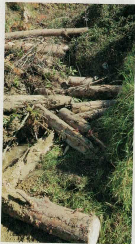
No, that's not a troublesome pile of forestry slash: these logs were carefully placed in the channels to slow water, reduce erosion and cause sedimentation build up, fending off the development of head cuts.
