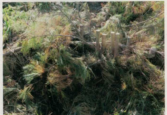
A completed post-and-weave leaky weir on an erosion channel.
