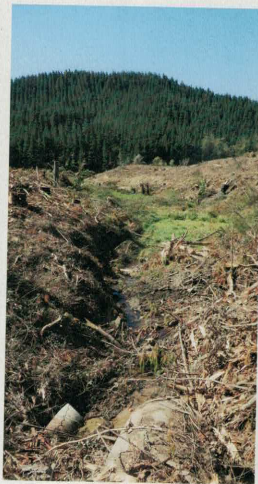
Before: the stream and the surrounding area is eroding significantly.
