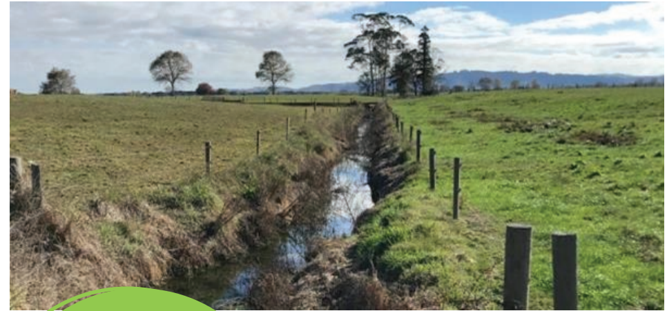
A section of trial drain before planting, Fences stayed where they were. 2022. Photo: WRC
